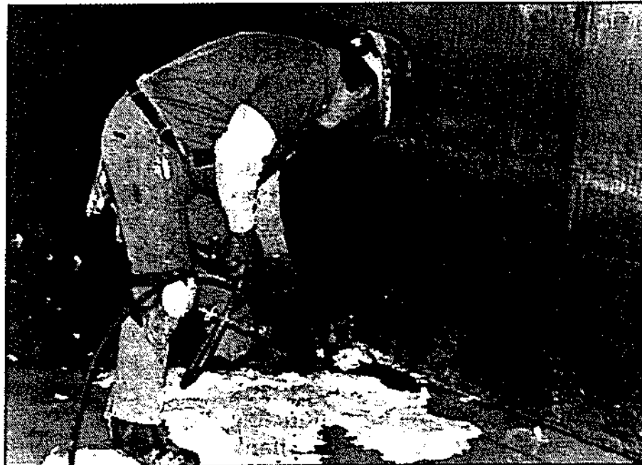
Liquid grout injected into cracked concrete reservoirs keeps the drinking water in and the groundwater out.
